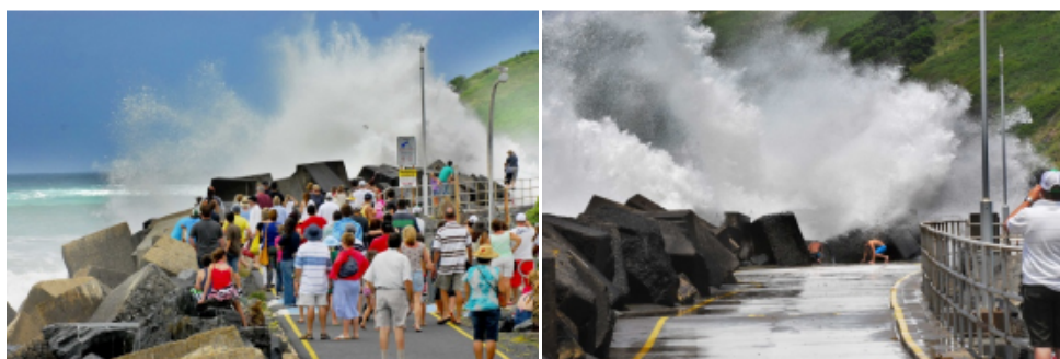
Figure 2: Coffs Harbour North Breakwater showing section subject to wave overtopping (sourced from MHL, 1994)
